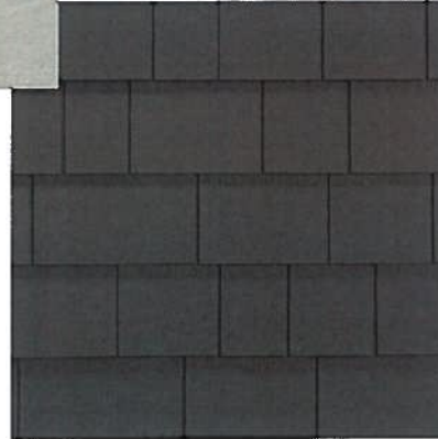
5. cement board staggered edge
