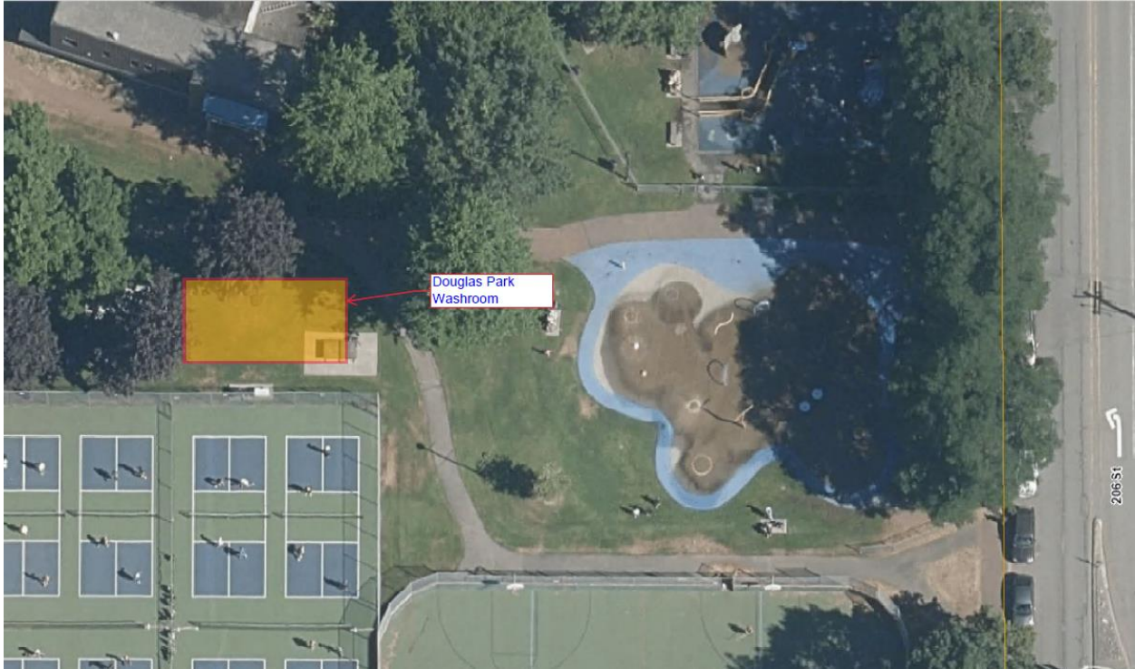
Project Location: Douglas Park Public Washroom (20550 Douglas Crescent)
