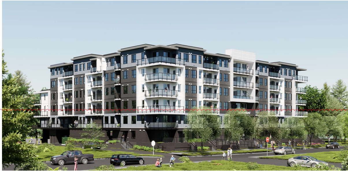
SOUTH/WEST CORNER OF DEVELOPMENT
