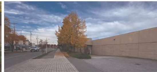
10 - 203 STREET, LANGLEY MALL ON THE RIGHT
