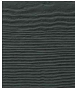
7- Fiber Cement Panelling with Reveal Color to Match: James Hardie_ Iron Gray
