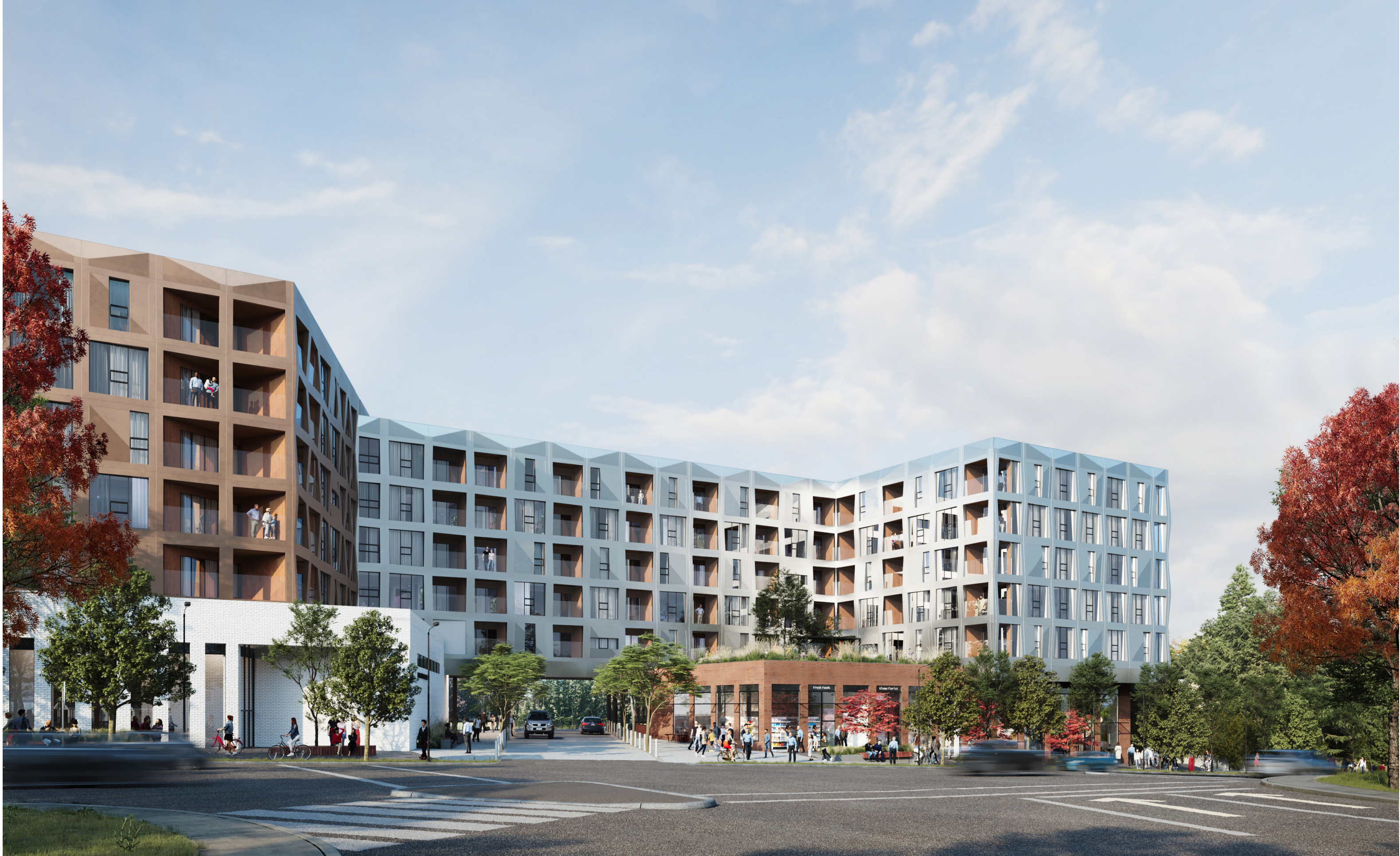
View looking west toward 200 Street, from Grade Crescent
