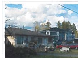
THE TWO PROPERTIES IN THE CURRENT CONDITION WITH A PRONOUNCED DITCH ALONG 55A AVE.
