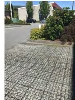
ENGINEERED BASE WITH GRAVEL AT VISITOR PARKING
