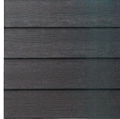
3. cement board horizontal lap siding
