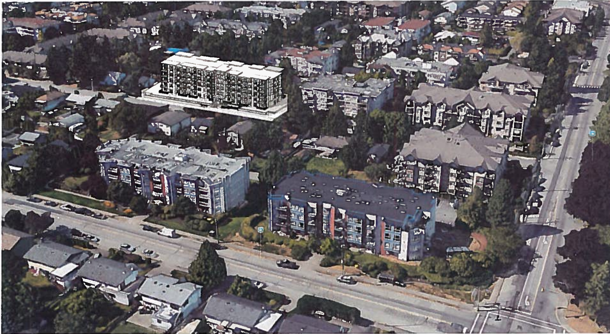
Aerial view at north east
