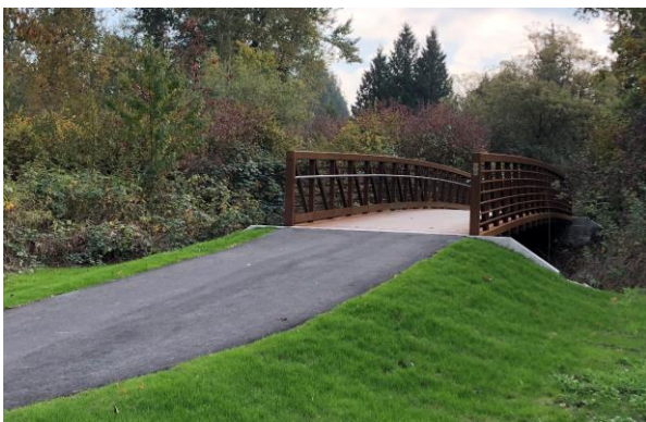
201A St Pedestrian Bridge (installed in 2018)
