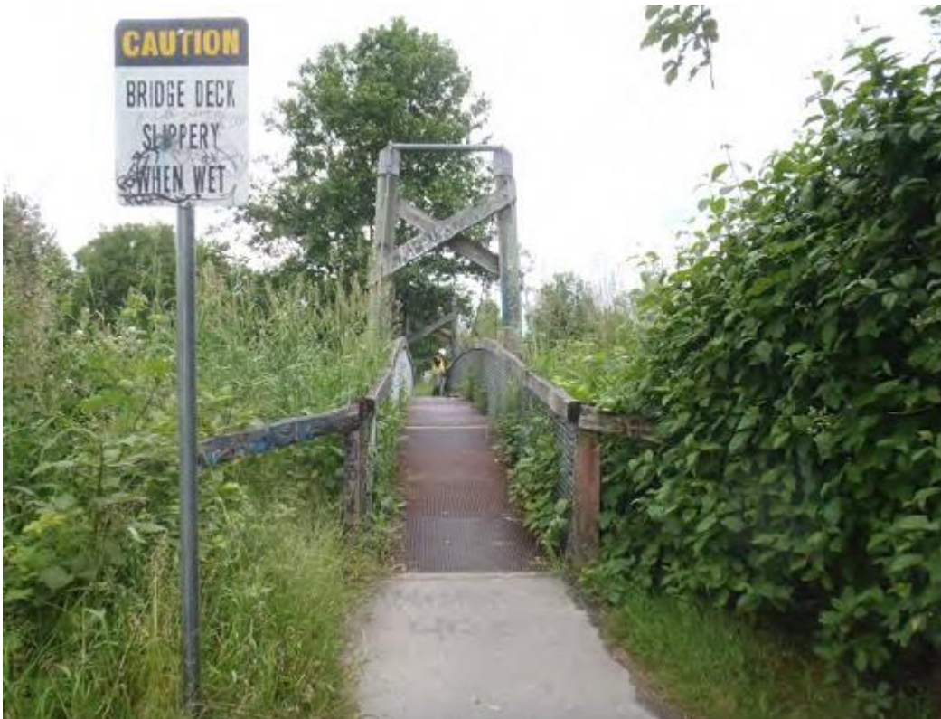
206A St Pedestrian Bridge
