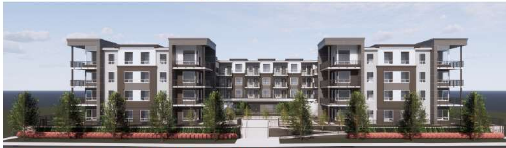
lincoln apartments - keystone (under construction)
