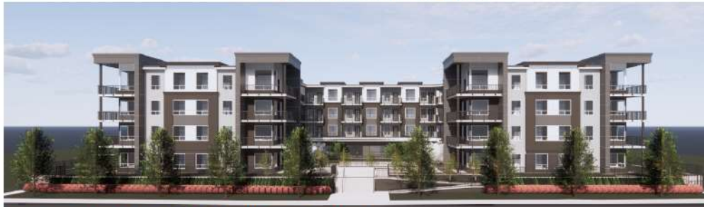
lincoln apartments - keystone (under construction)
