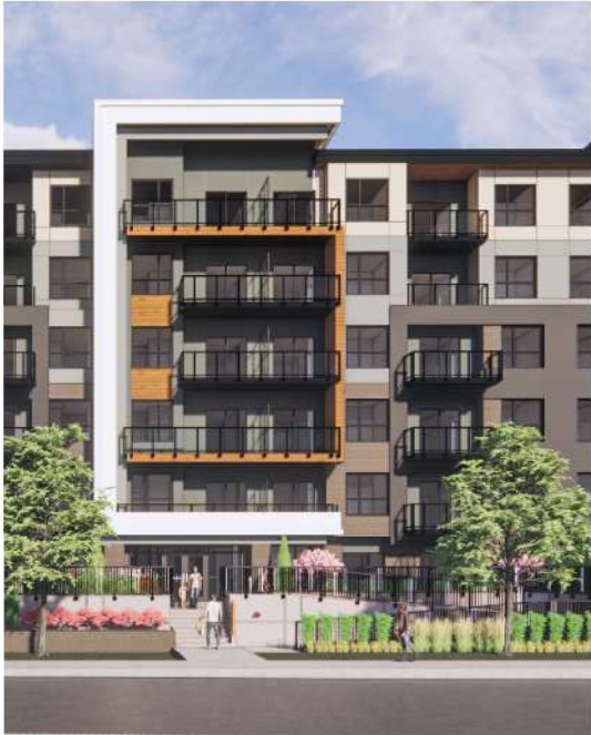
main building entrance
