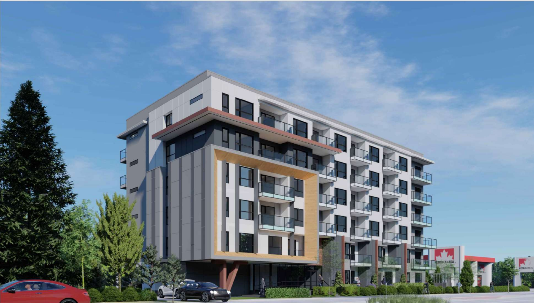
NORTH EAST CORNER
