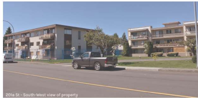
201a St - South-West view of property
