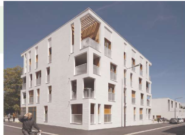
Case Study Social Housing in Tours Atelier du Pont Tours, France 2019
