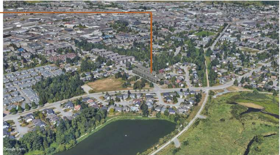
aerial view looking n/w
