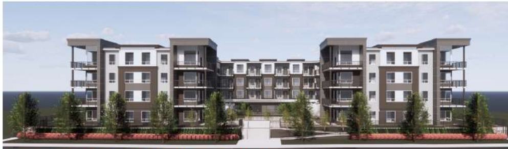
lincoln apartments - keystone (under construction)
