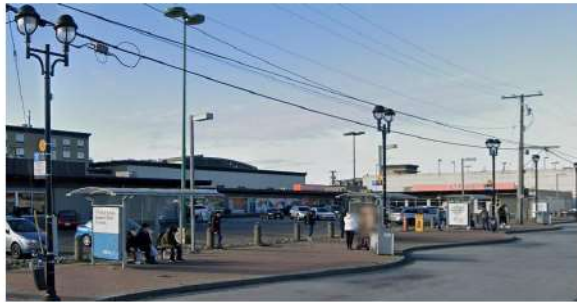
bay 4 transit station
