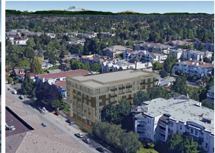
③ STREETScape VIEW ALONG 54A AVENUE
