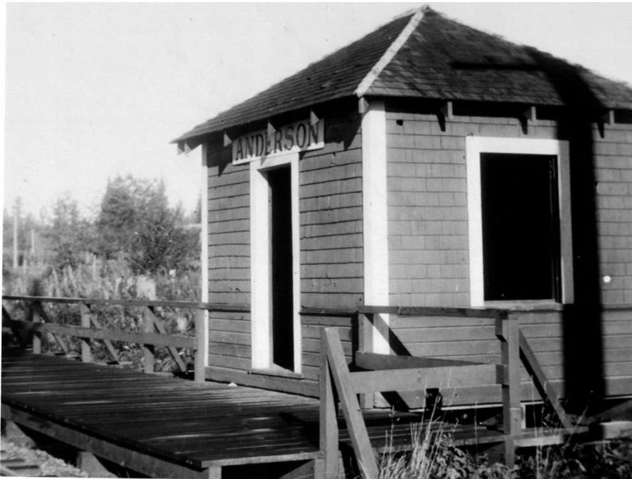
BCER Anderson station at 192 nd Street and the BCER pathway in Surrey.
