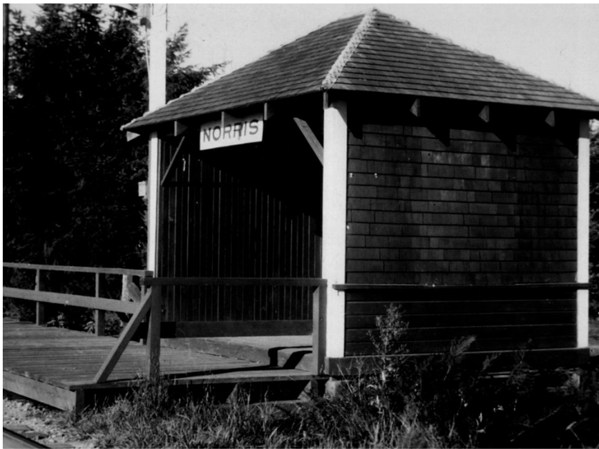
BCER Norris Station, formerly at Glover Road and Mufford Crescent, has been fully restored and is now located at the Leaf House property on 272 nd Street. The extension of Mufford Crescent to connect with the redesigned Glover Road has eradicated the original Norris Station site.
