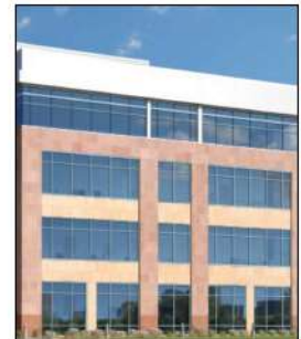
10 - Glass: Guardian Glass Color to Match: SNR43 Crystal Gray (Only on south elevation)
