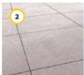
2 Cast-in-place concrete pavement
