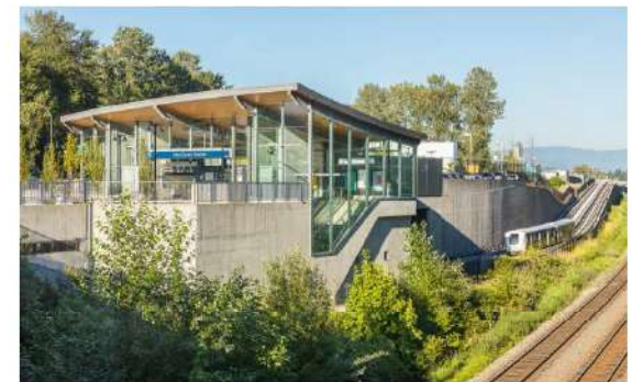
Inlet Centre Station
