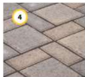
4 Unit paver pavement
