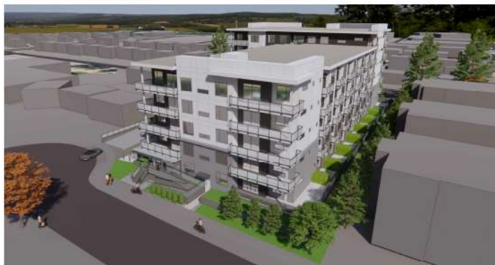
AERIAL VIEW FROM SOUTHWEST
