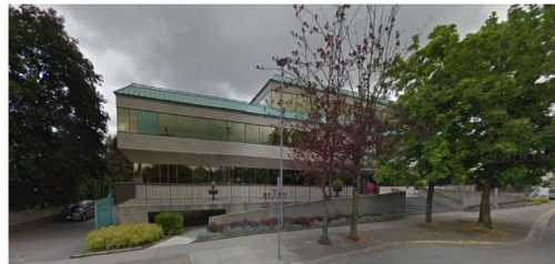
existing building looking south
