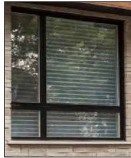
1 - Double Glazed Windows Color to Match: Benjamin Moore Black Ink_2127-20 Glass: Clear
