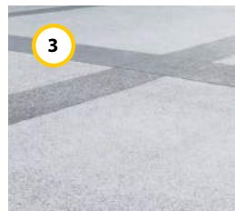
3 Exposed aggregate concrete bands
