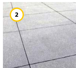
2 Cast-in-place concrete pavement
