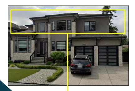
3<sup>rd</sup> storey floor area = 80% of storey below; 1.2 m. stepbacks (front/side)
