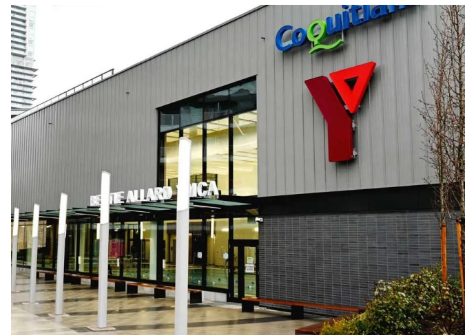
Park-and-ride parking spaces secured by City of Coquitlam as part of Coquitlam Bettie Allard YMCA development by Burquitlam Station
